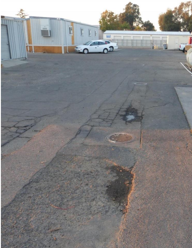
Failing AC paving within the Public Works Yard
